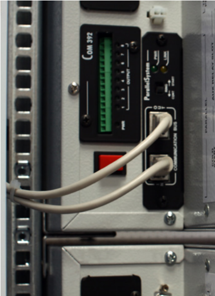
Parallel configuration and programmable relay contacts board.
